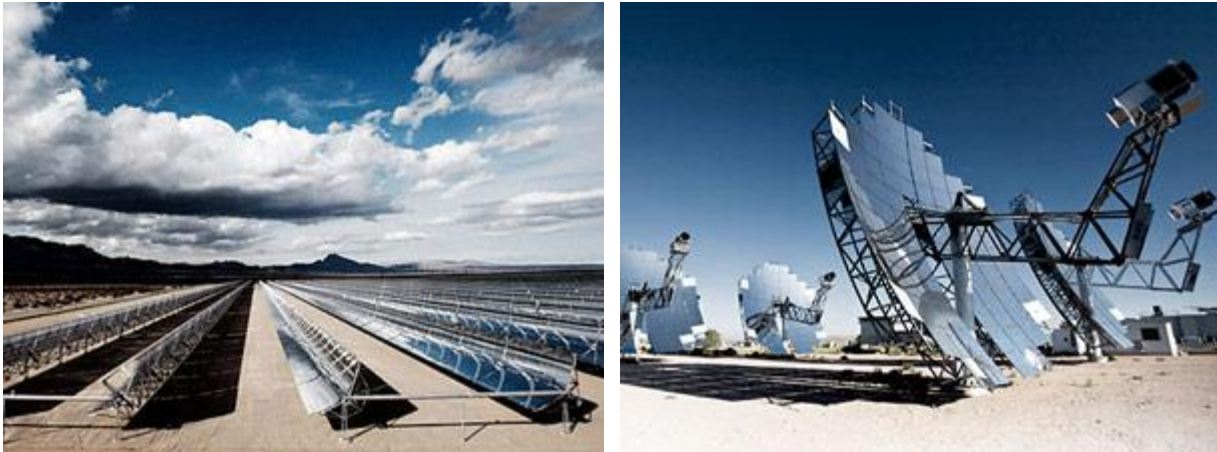
Figure 7 Parabolic trough and solar dish CSP (Hutchinson, 2008).
