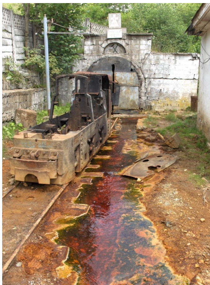
Figure 17 – Adit 714 releasing contaminated water.
