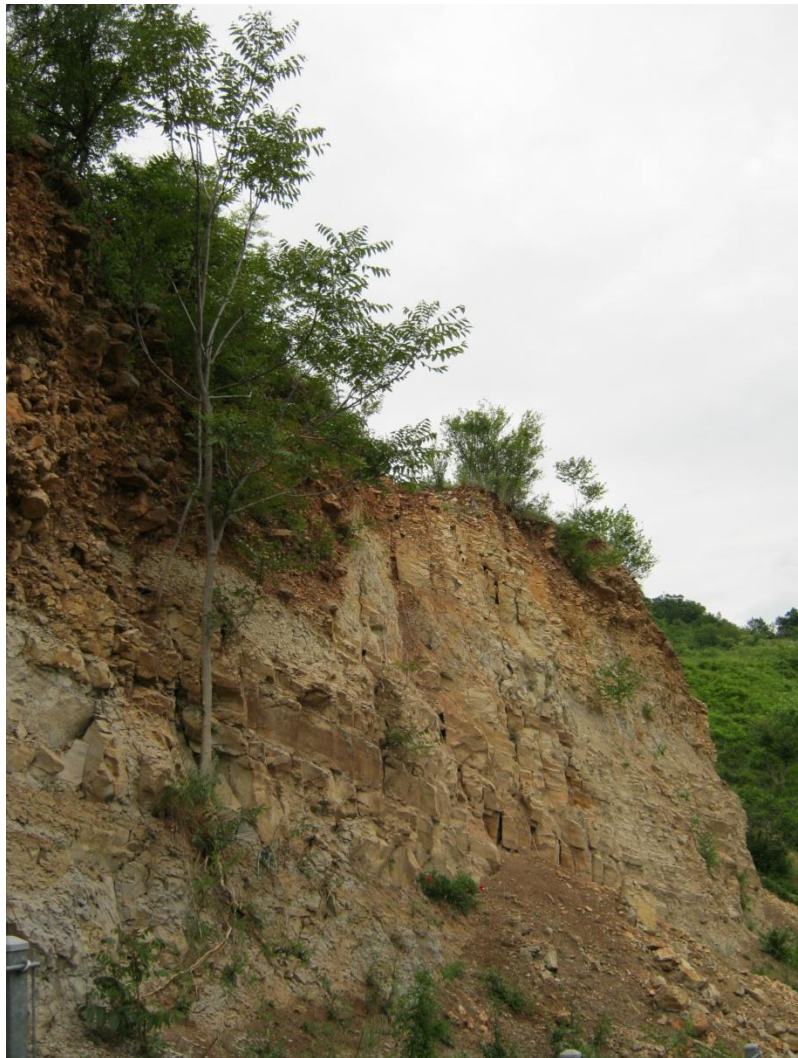
Some of the observed slopes are in an extremely unstable conditions and are in imminent possibility of collapse, possibly along the planes further weakened by weathering and burning.
